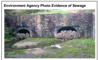
**Note:** Sewage rags on culvert outlets are positive evidence of sewage discharge to the stream.
